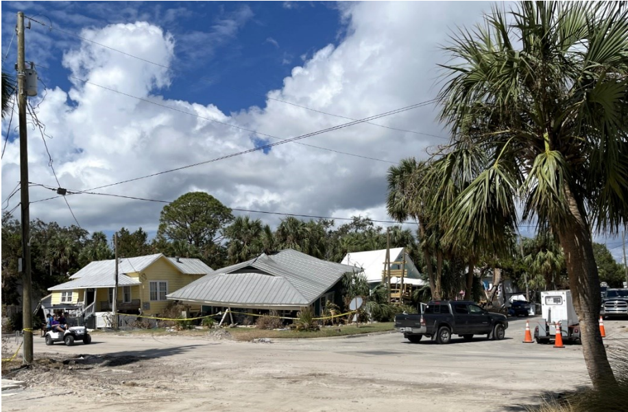
Figure 1. Extensive damage caused by Hurricane Helene in September 2024.
