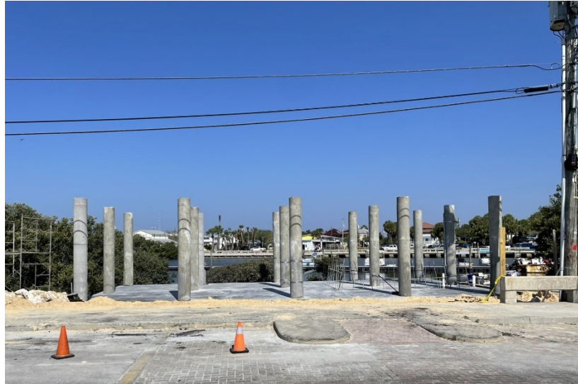
Figure 4. Business recovery work at Dock Street.
