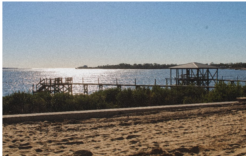
Figure 3. 6th Street Pocket Park. Image, edge consolidation with bulkhead.
