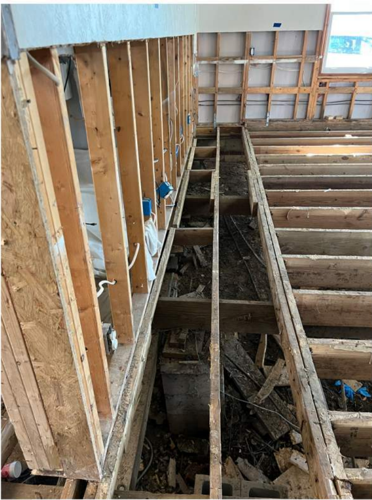
Framing between Renovation Phases
