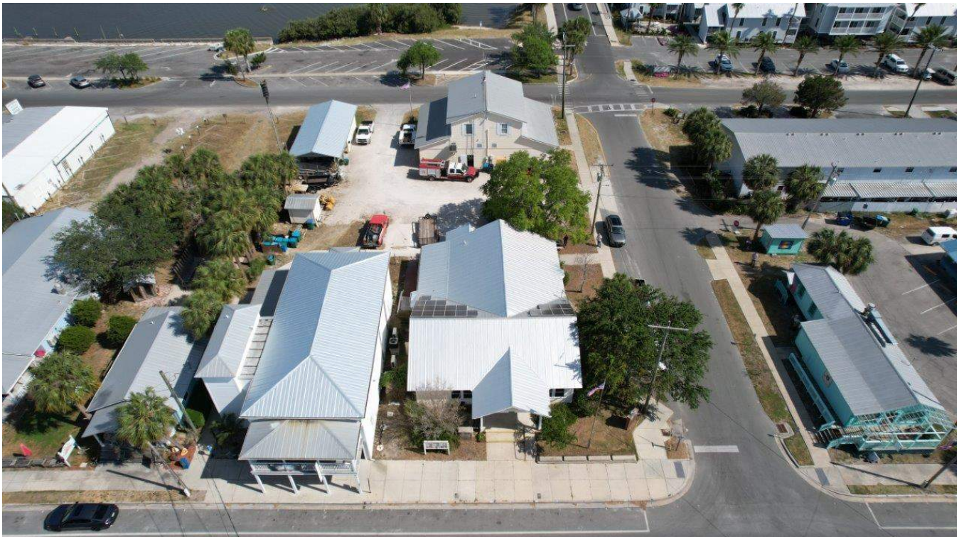
Aerial View of the Site and Surrounding Context
