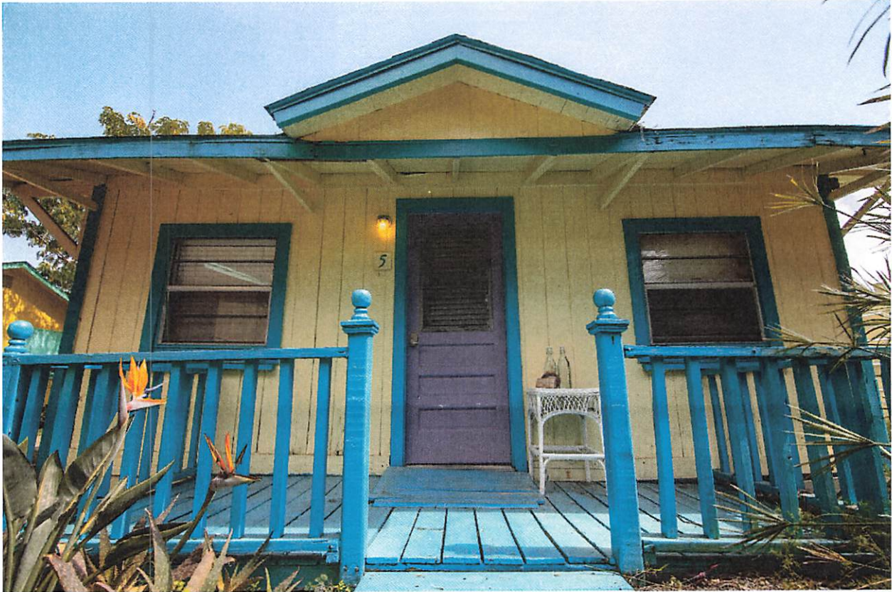
Example of the Cracker-style architecture: long eaves, bid deck, oppositional windows, open crawl space underneath.
