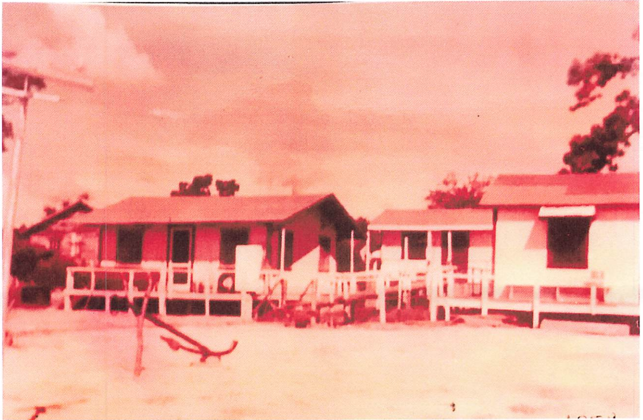
This 1954 shot shows the back cottages, and their wrap around decks and overhanging eaves
